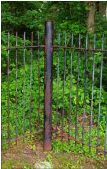
Figure 181. Southeast corner of the cemetery and replacement fence post.
