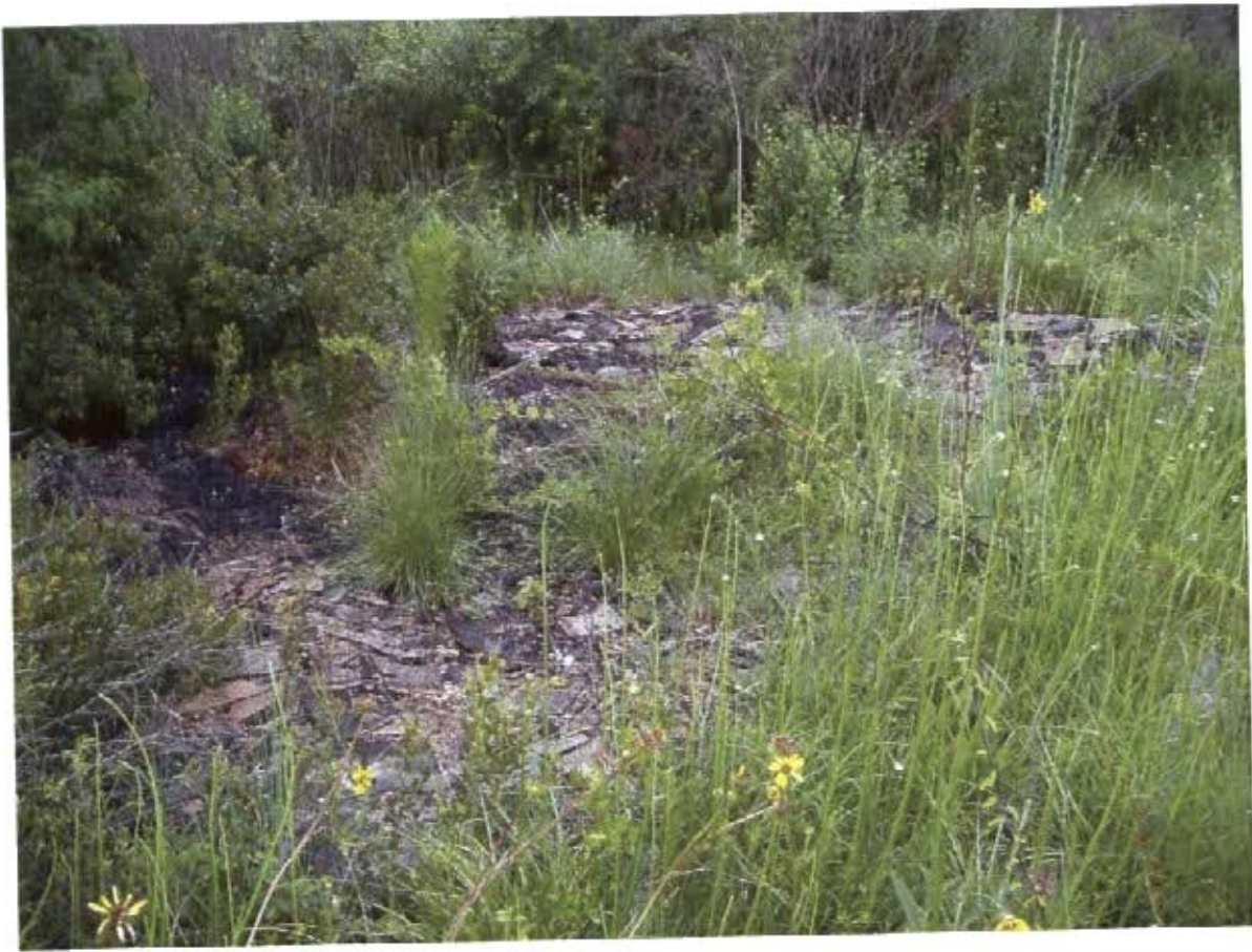
Photograph 5 – View of shingle debris pile observed in central portion of property.
