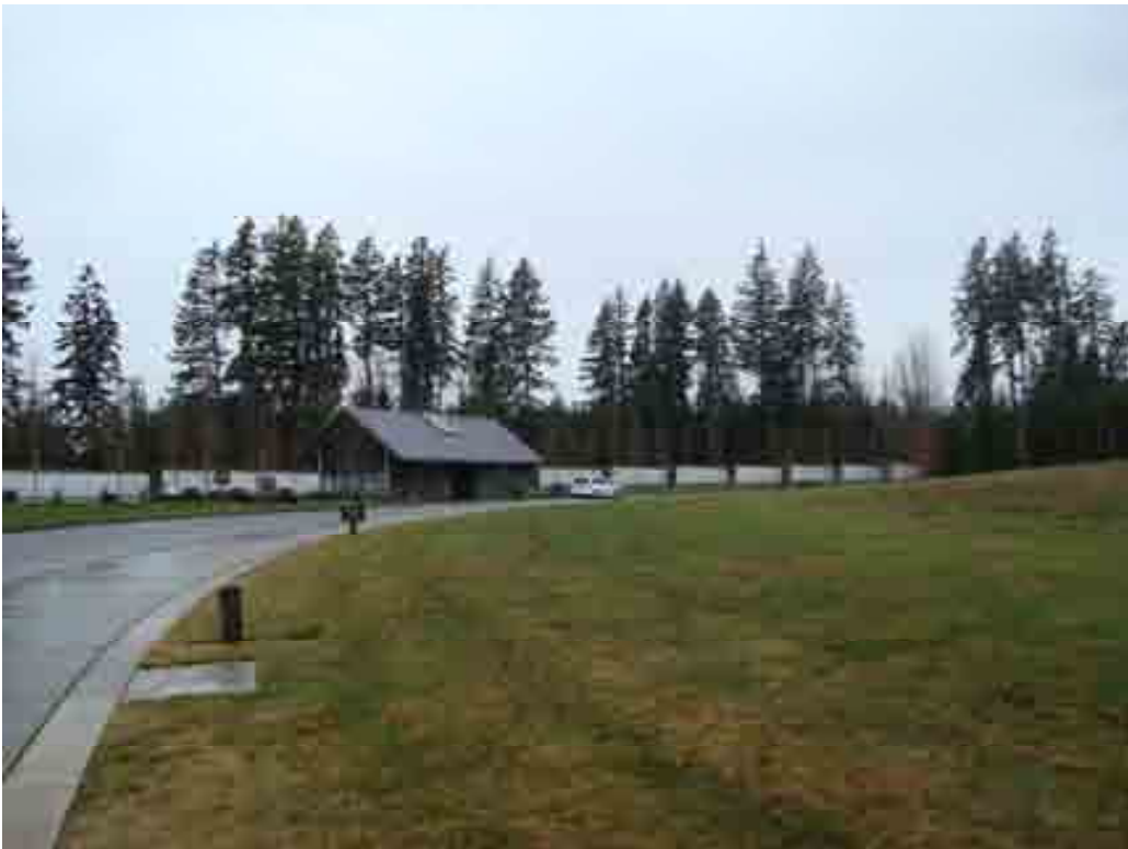
Photo 2 – View of the visitor center and main roadway located in the southern portion of the site, facing west-northwest.
