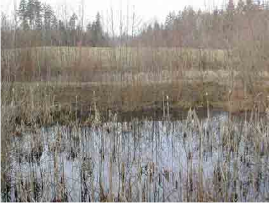
Photo 9: View of stormwater management area located in the southeastern development area, facing northwest.
