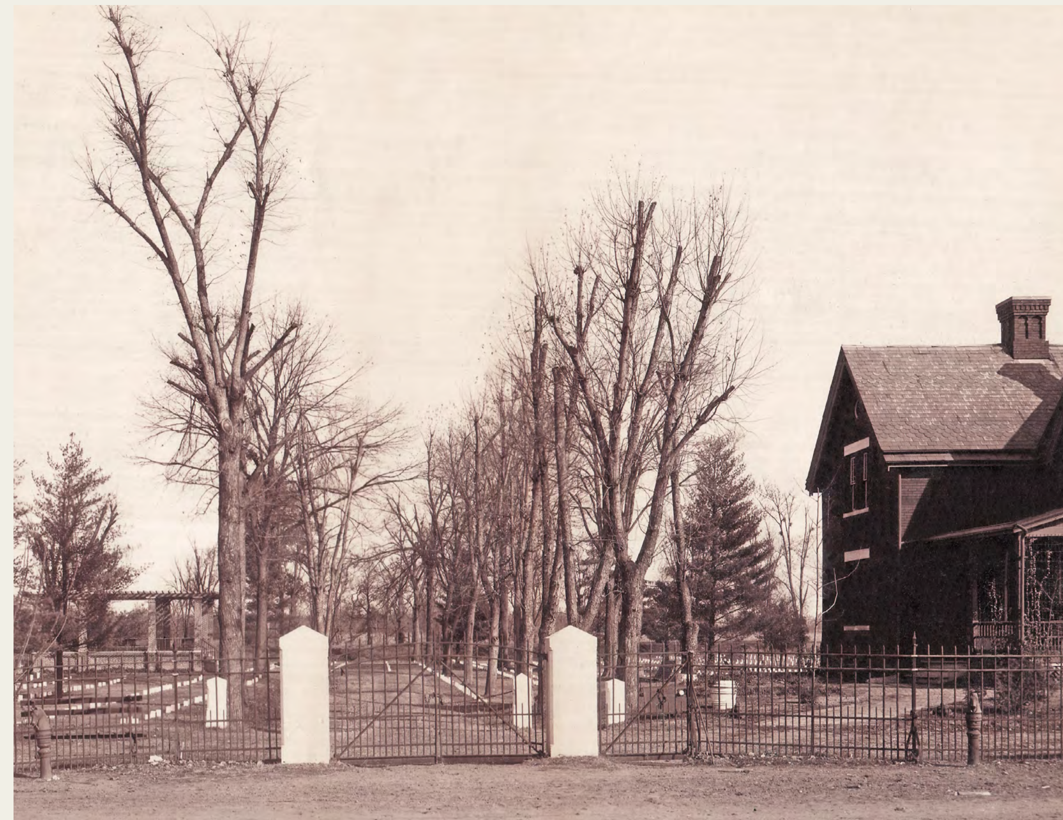
View of cemetery entrance with rostrum (left) and lodge (right), 1903. National Archives and Records Administration.
