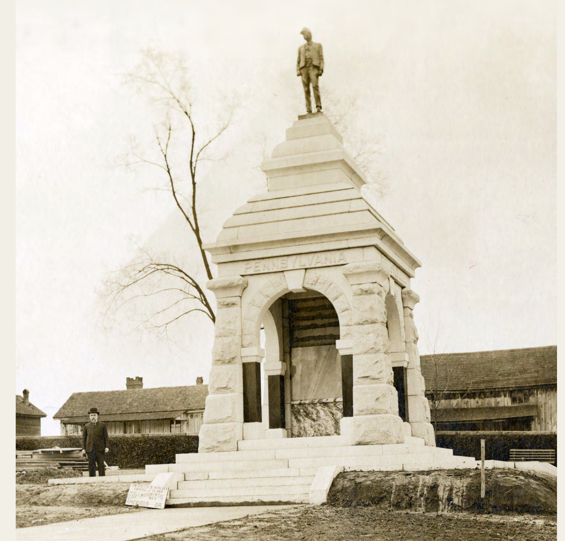
Pennsylvania Monument under construction. National Cemetery Administration.
